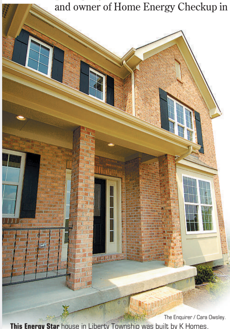
This Energy Star house in Liberty Township was built by K Homes.
